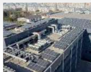
上海嘉定总部176kW分布式光伏电站 Jiading HQ Building 176kW PV Power Station
